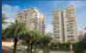
Shalimar Gallant, Mahanagar, Lucknow UPRERAPRJ3168
